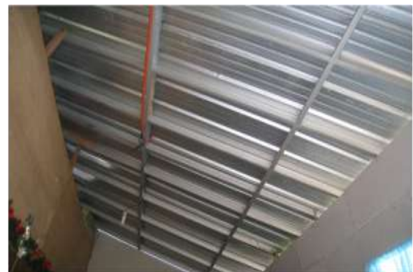
Figure 3.8 The hardiflex steel frame
