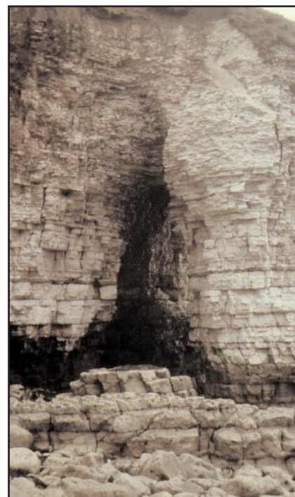
Figure 9: Taken only three months after the arch collapsed in 1984. Most of the debris has already disappeared
