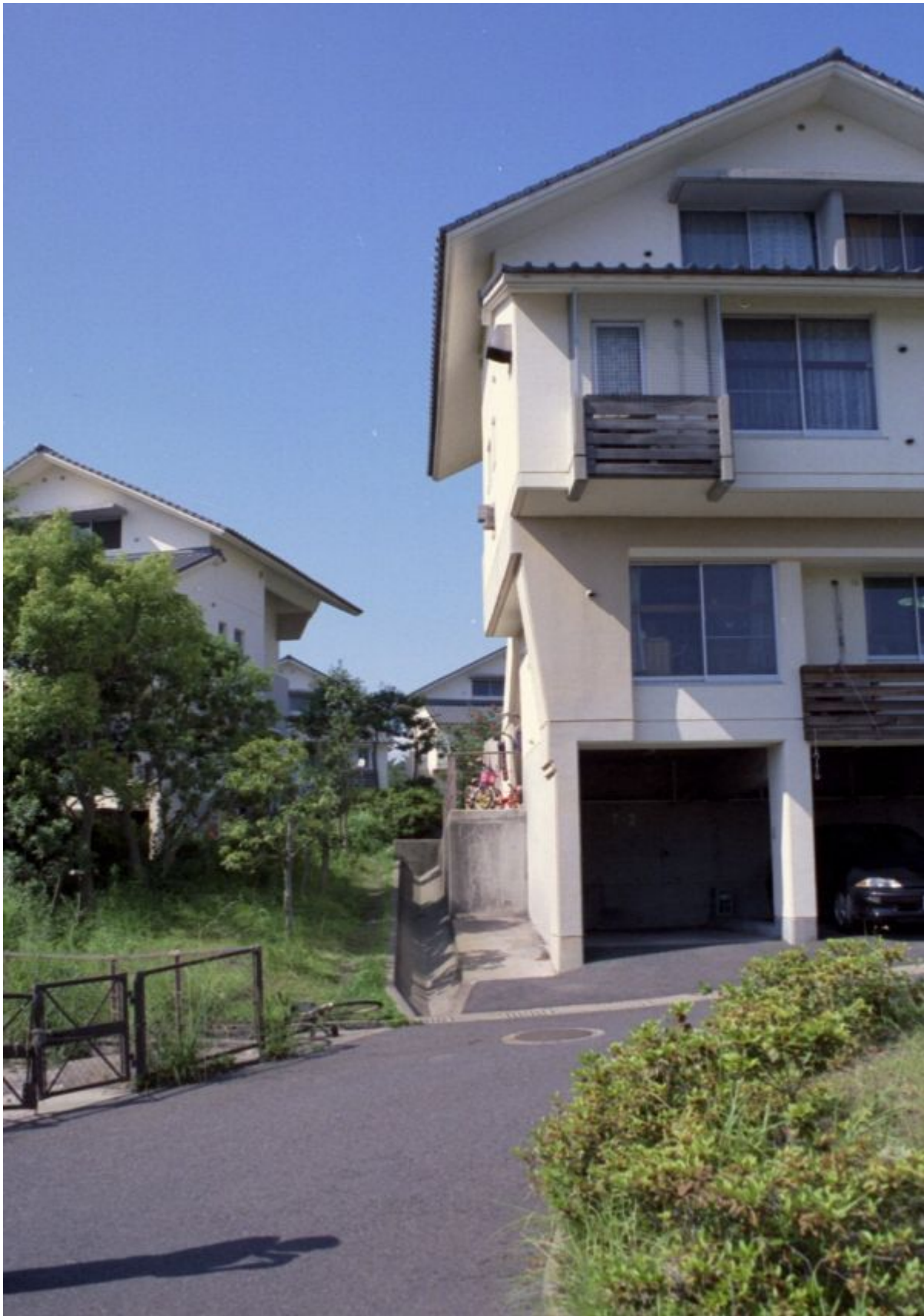
Figure 6. An example of urban design used to mitigate the effects of ash fall in Kagoshima, Japan. The design of the housing includes gutter-free roofs (which have a storm water channel located directly beneath), ash-resistant tiles, heavy-duty rubber window and door seals (to aid air tightness to prevent ash entering houses) and large overhanging roofs over balconies (Photo: David Johnston).
